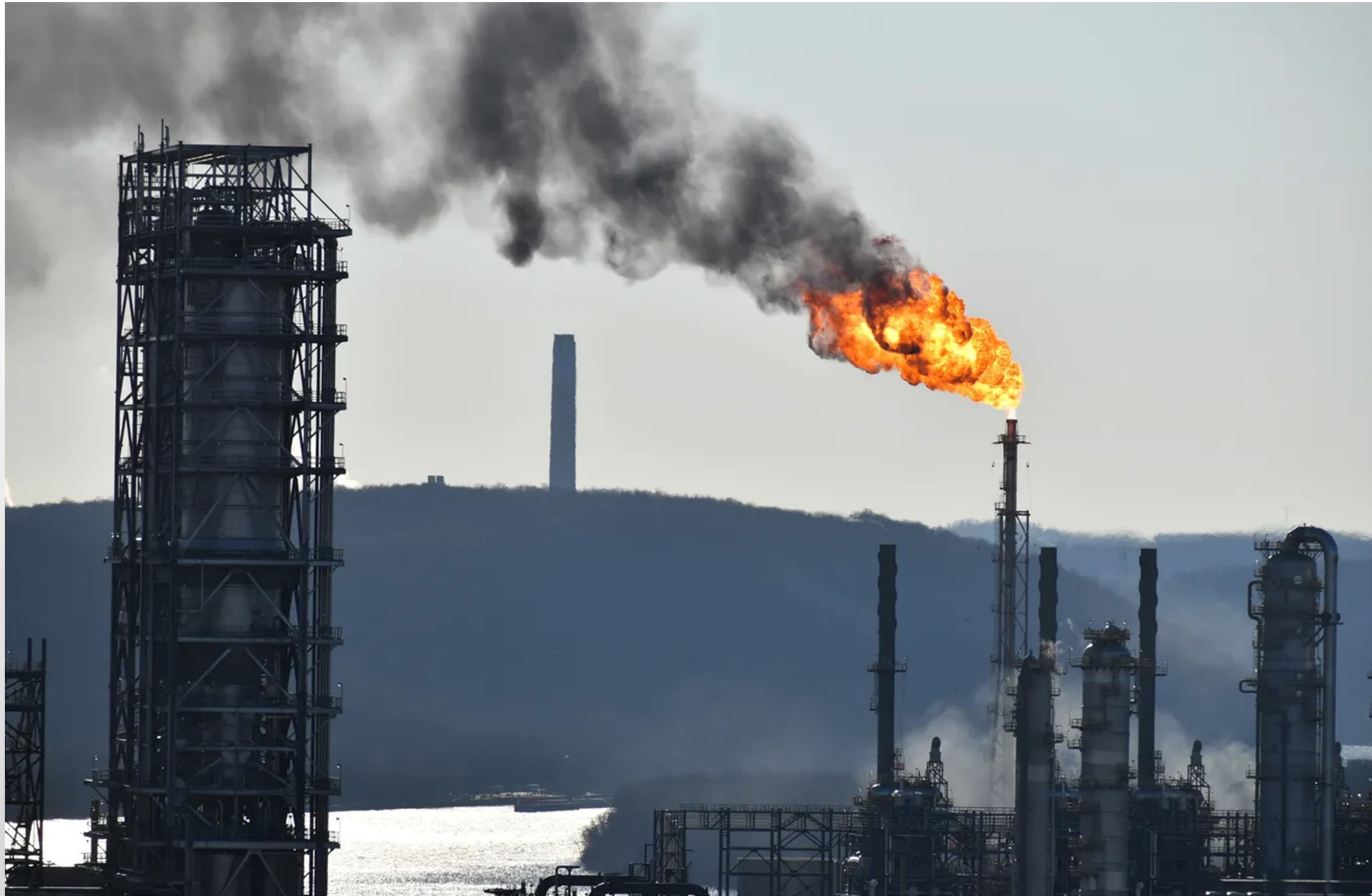
Shell's elevated flare seen over Potter Township on Feb. 13, 2023. Chrissy Suttles/BCT
